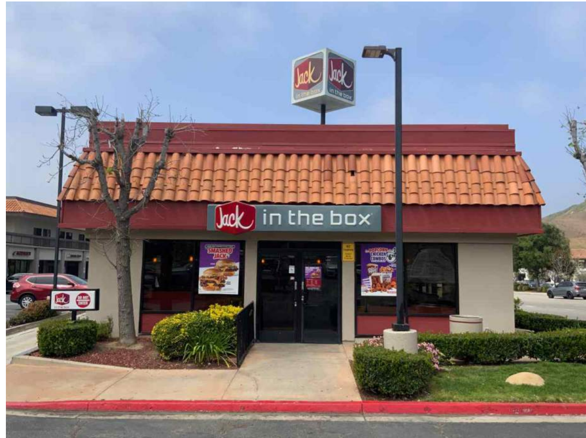
EAST ELEVATION: PHOTO OF EXISTING
