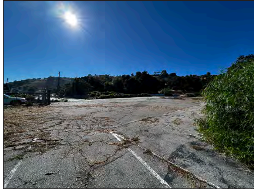
Photo 1B - Photograph of northernmost portion of the Survey Area showing existing paved parking area.
