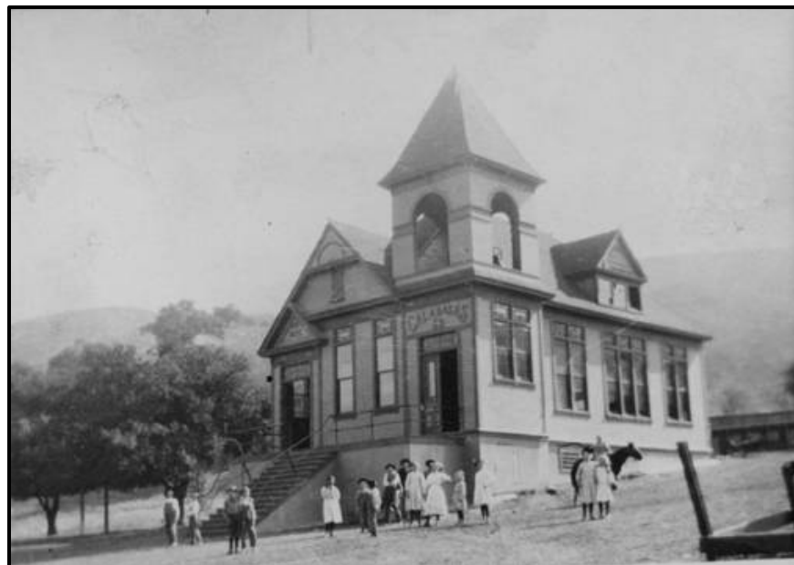
Figure 5: The 1890 Calabasas school, located immediately east of the Project property.
