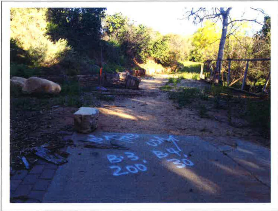
NEAR BORING B-4 LOOKING WEST TOWARDS BORING B-3
