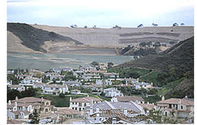
The Oaks of Calabasas - View of Homes Under Construction
