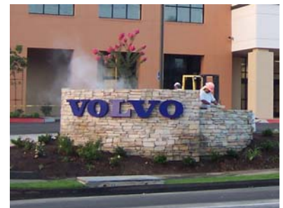
Calabasas Volvo— View of Monument Sign under Construction
