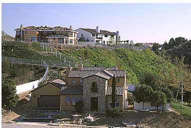
The Oaks of Calabasas - View of Homes Under Construction
