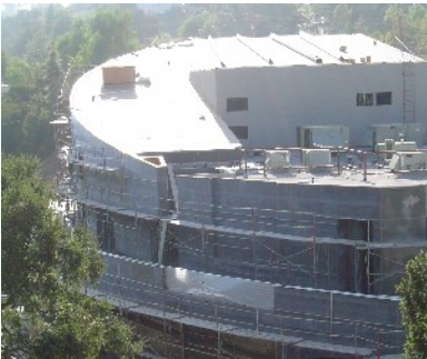
Viewpoint School— View of Performing Arts Center under construction
