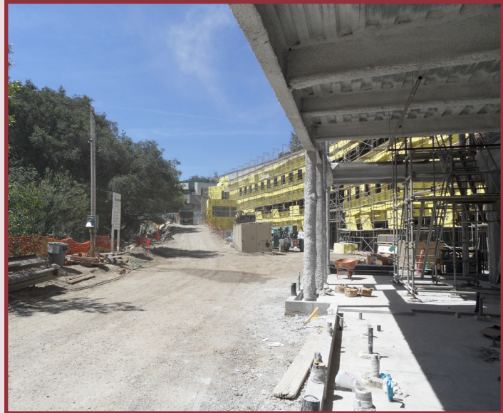
Construction of upper school building
